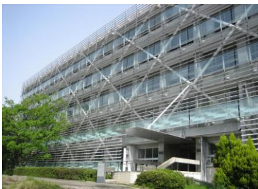
Seismic retrofit of aged building
